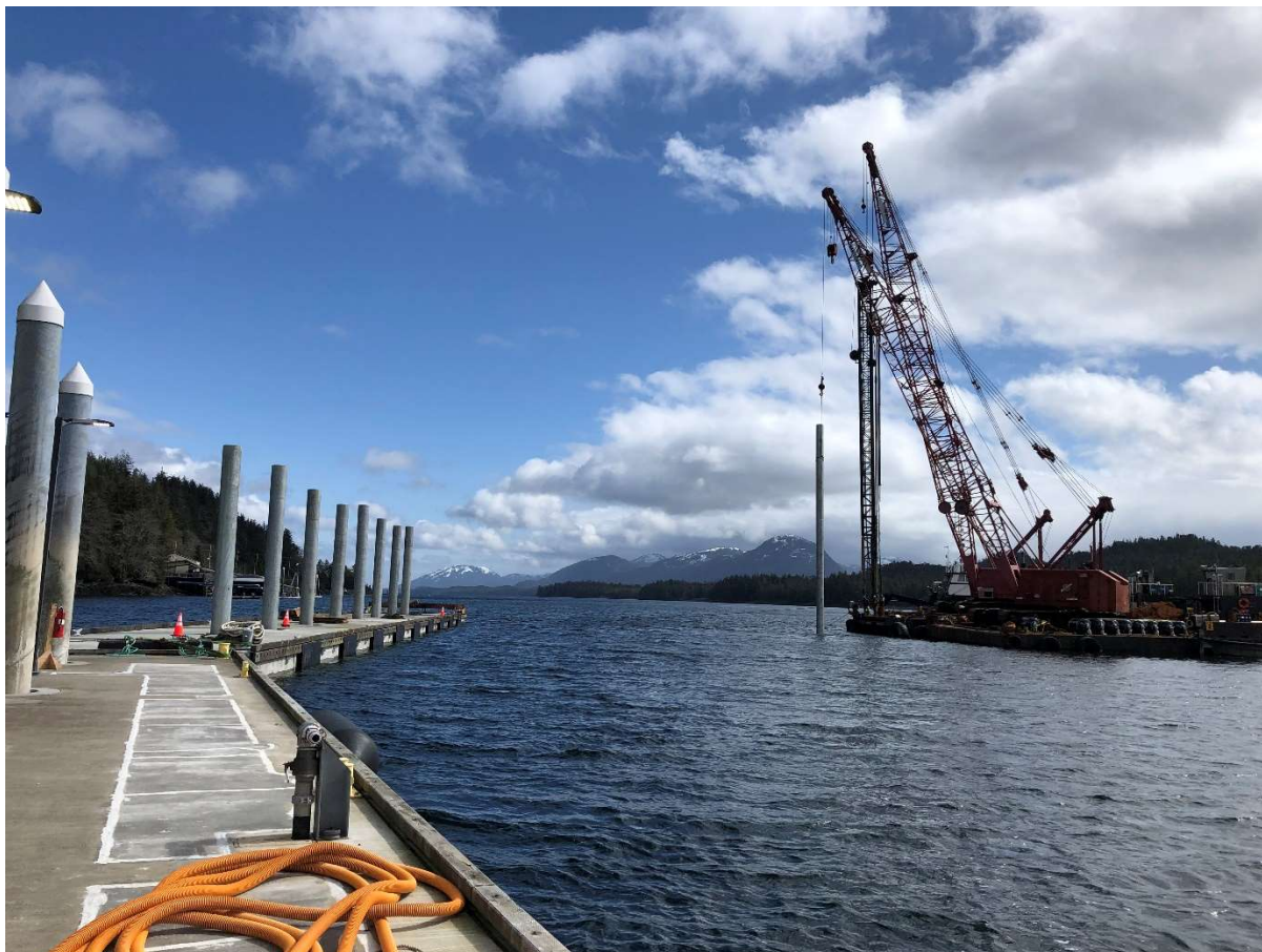
New floating dock with 9 th piling suspended from crane, 26 April 2023.
